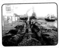
Sues Road isn't set for replacement for several years yet, so we felt it was time to try a different approach. We researched possible solutions and felt a French Drain System would best serve as a solution at the lowest
